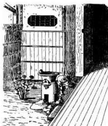
Fig. 237.—Verandah showing swinging closet for rain-doors, and also Chōdzū-bachi.
